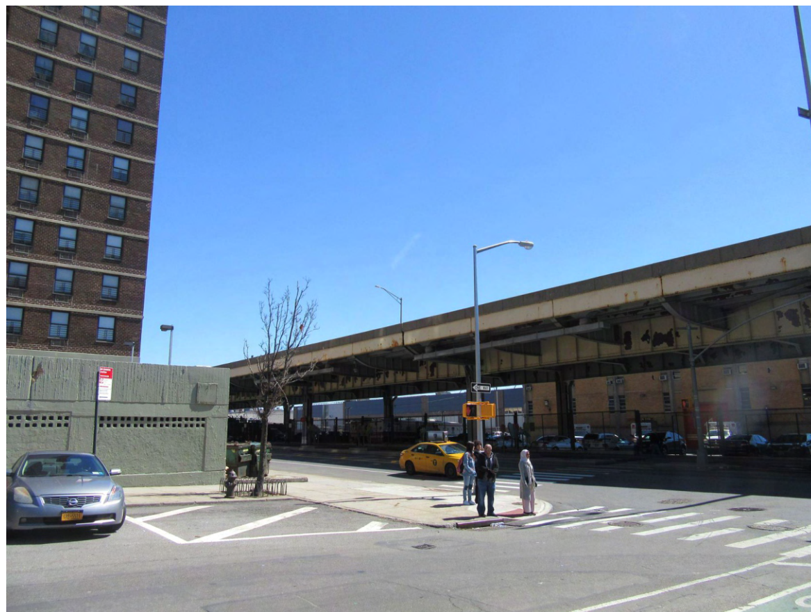
21. View of the intersection of Clinton Street and South Street facing southeast (Parcel 7 at far left).
