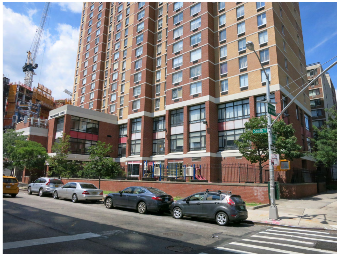
9. View of the Development Site facing northwest from South Street.
