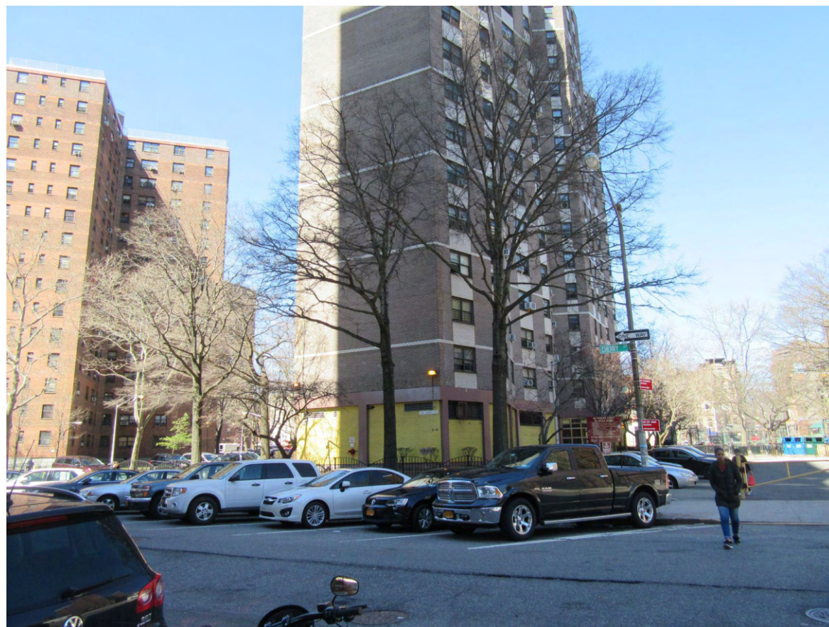
18. View of the north side of Cherry Street between Rutgers Street and Jefferson Street facing northwest.
