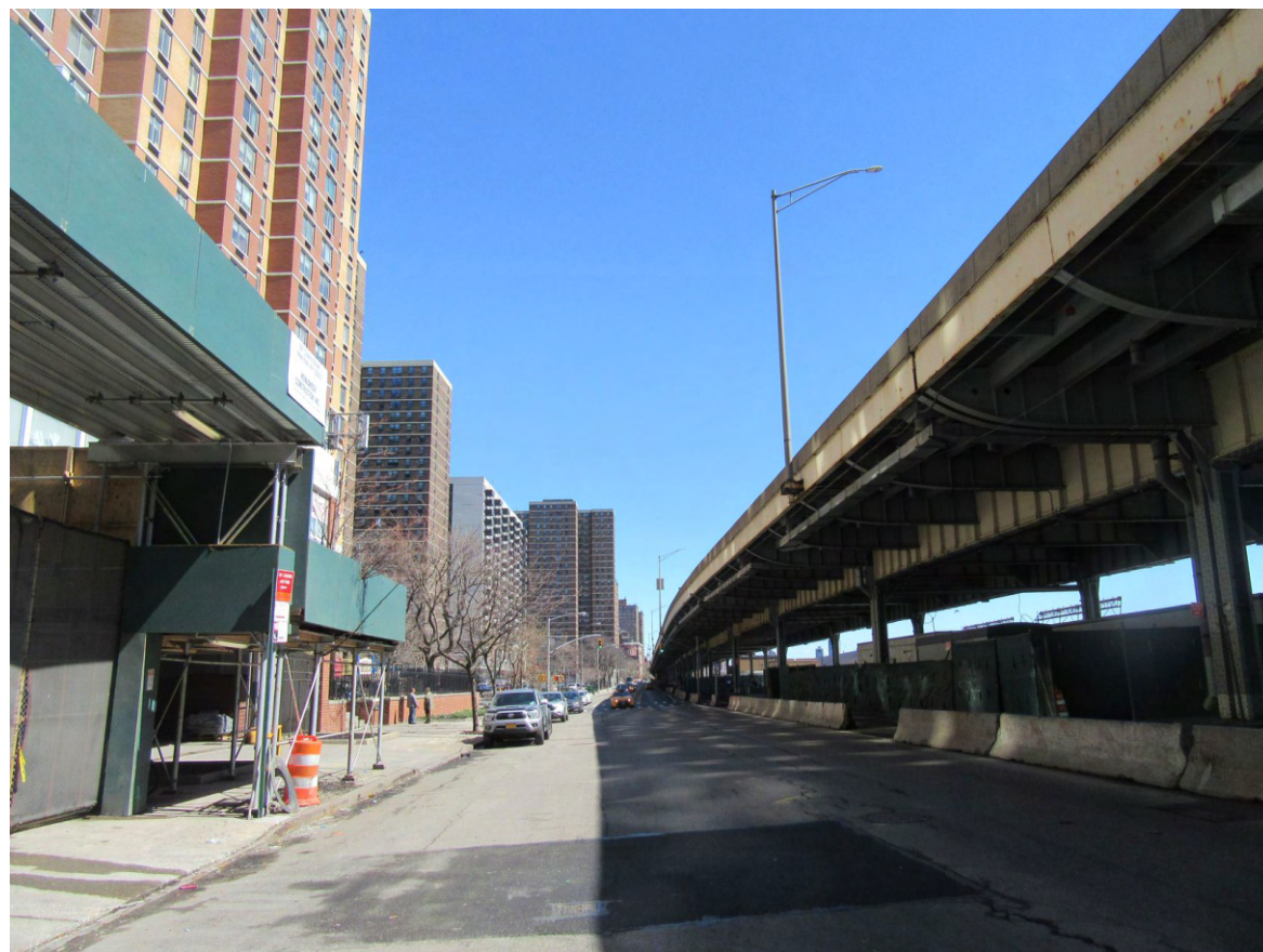
27. View of South Street facing east toward Rutgers Slip (Development Site at left).
